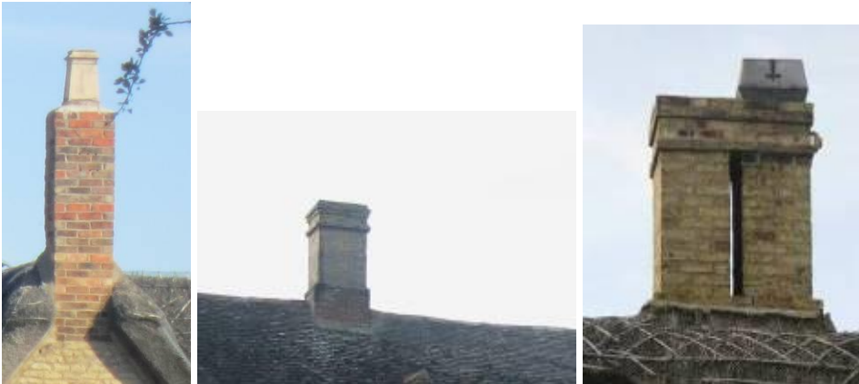
Brick chimneys inserted in to 17 th and 18 th century buildings
