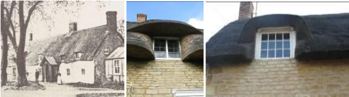
longstraw thatch roofs with hooded and eyebrow dormers
