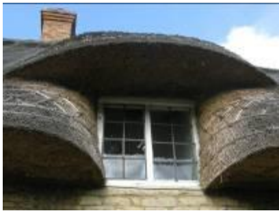
Lights made of wrought frames and leaded lights, Waterend Cottages
